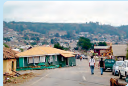
Pelluhue after the earthquake.
